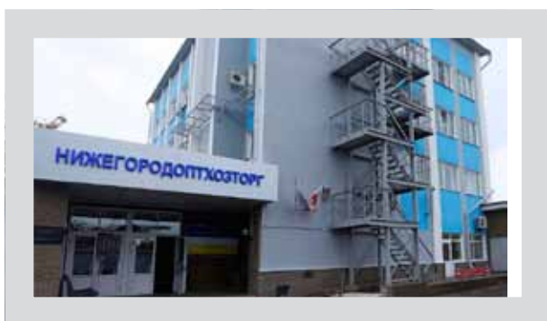
NOHT, reconstruction of the building
